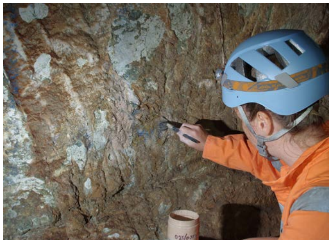
Figure 11 Covering graffiti by dabbing on a slurry of ground limestone and potters clay.
