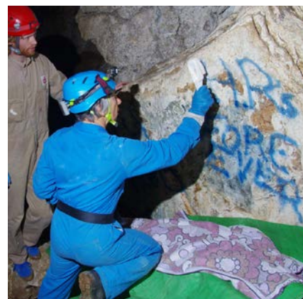
Figure 6 Drop sheets and towels are used to capture runoff water and paint fragments.
