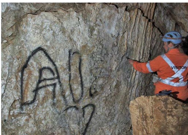
Figure 12 Working on a large area of graffiti that was sprayed onto a delicate and flaky surface.
